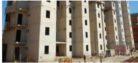
U \sim 3.5 \text{ W/m}^2\text{.K} Monolithic concrete wall
