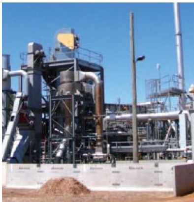
Biomass-fired power plant
