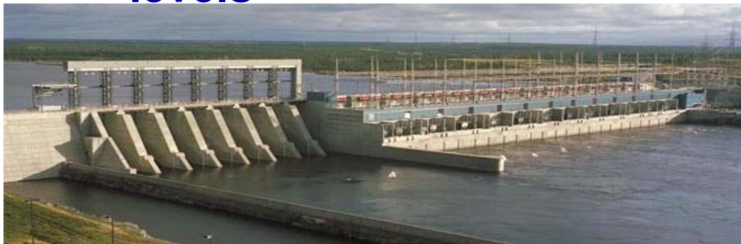
HQ Hydro facilities Baie-James, Canada
