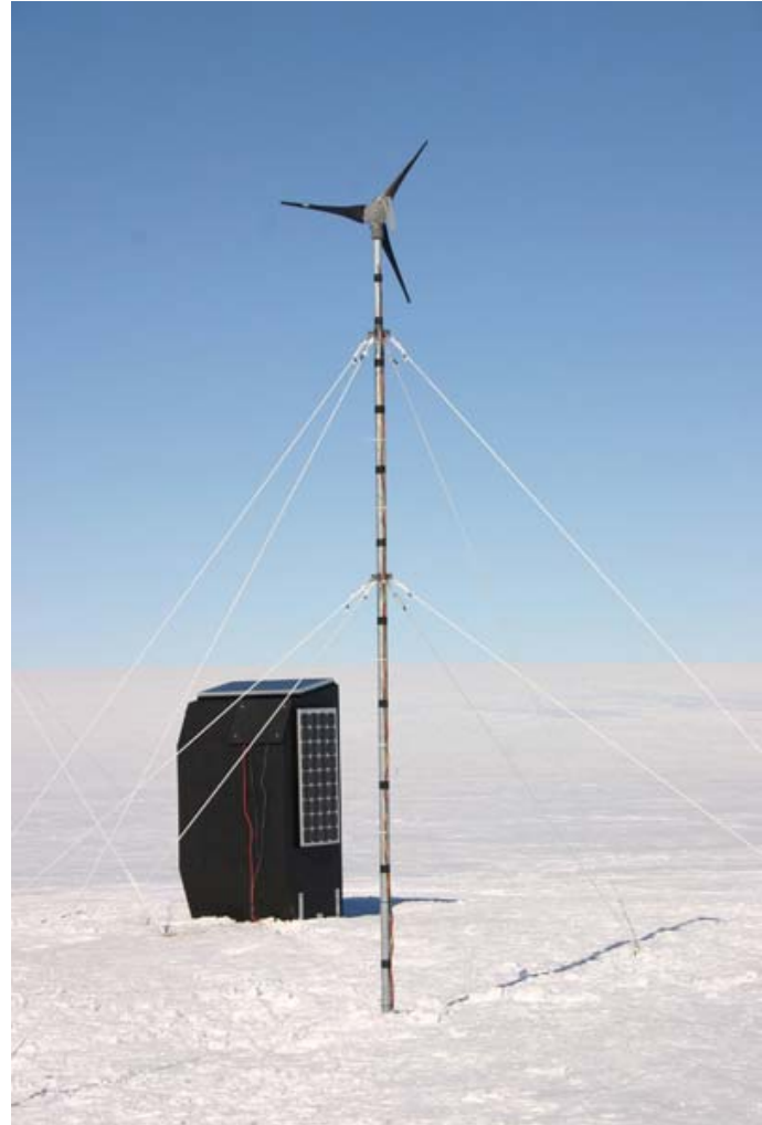
Mobile Base Station at SANAE in Antarctica powered by renewable energy
