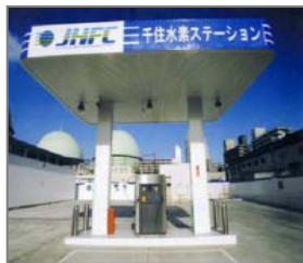
Hydrogen Fueling Station
