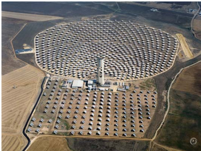
The PS10 solar tower plant being completed by Sanlúcar SA (Abengoa), Seville (Spain)
