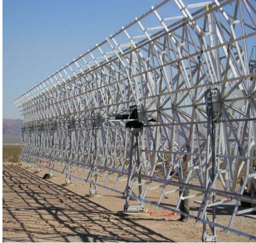
The Nevada Solargenix Solar One solar troughs take shape
