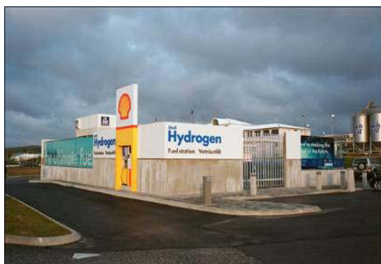
Shell Hydrogen Fuelling Station, Reykjavik, Iceland
