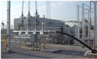
On 8 August 2006, a Southwire-NKT collaboration began demonstrating a prototype HTS cable (3 kA, 13.2 kV) of new design on the grid in Columbus, Ohio.
